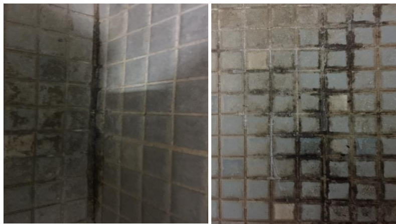
Figure 1: Stachybotrys chartarum in public bathroom
