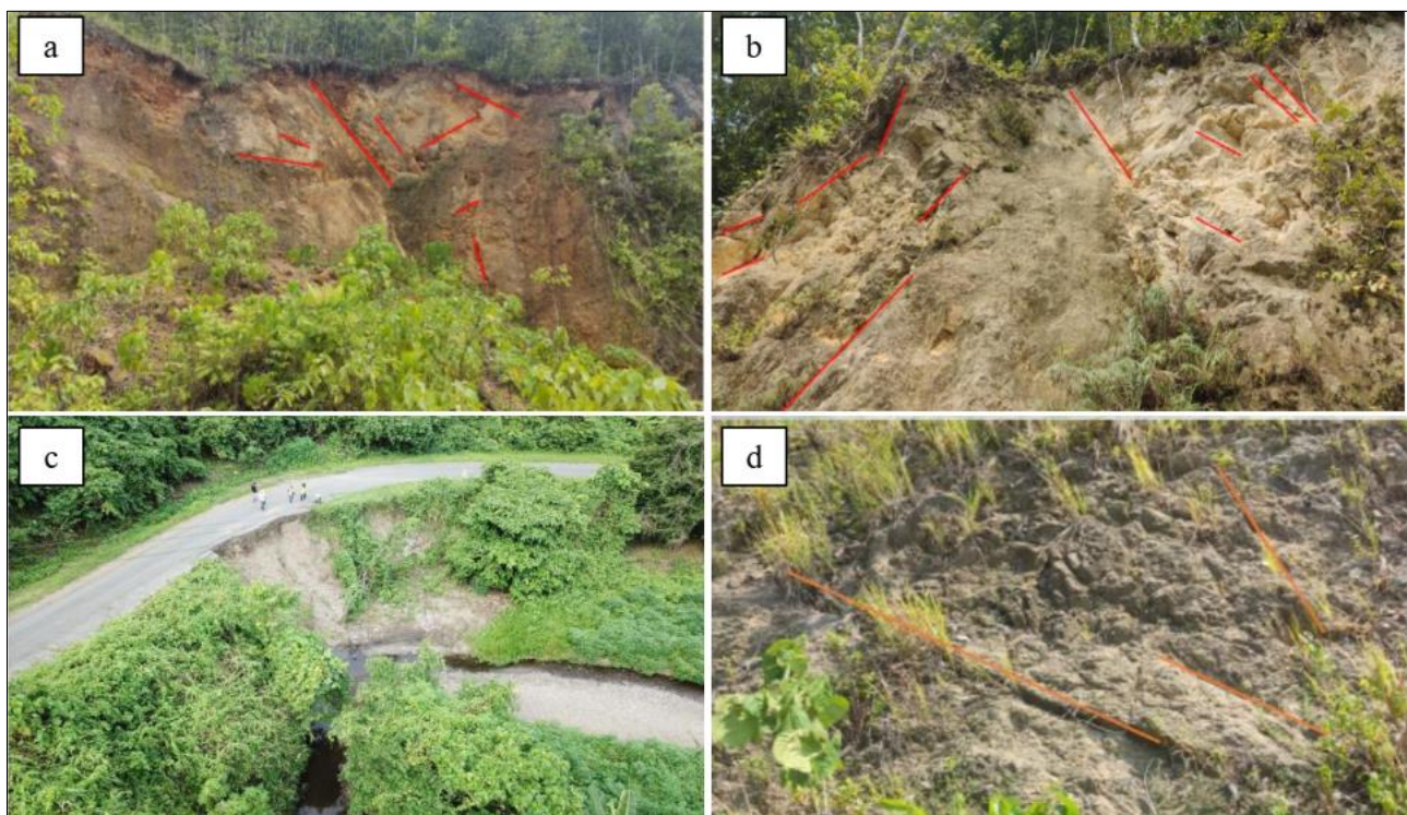
Figure 2: Types of landslide in research site (a) rock collapse at section 61-021-001-A (b) rock collapse at section 61-021-001-B (c) fill collapse at section 61-0233-001-B (d) fill collapse at section 61-0233-002-B.
