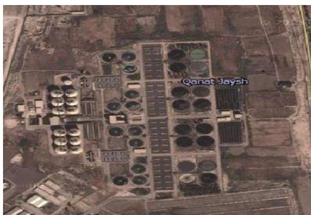
Image captured by Google earth 2010 for Rustumihia WWTP
